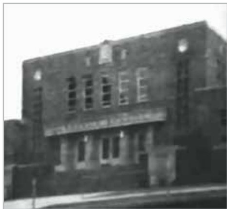
1948 | Lawrence Community Center
